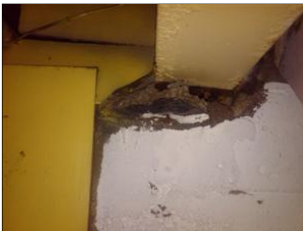
Repair Shims under Beam
