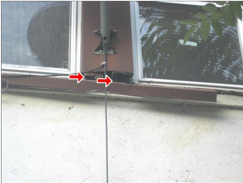
I. Picture 3 rot / damaged framing
