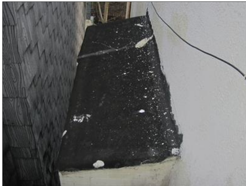
D. Picture 2 aged / deteriorated lower roof
