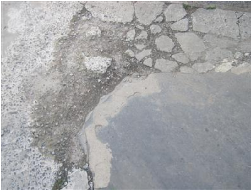
C. Picture 6 damaged sidewalk
