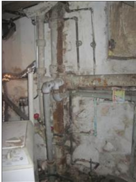
B. Picture 2 leaking corroded drains
