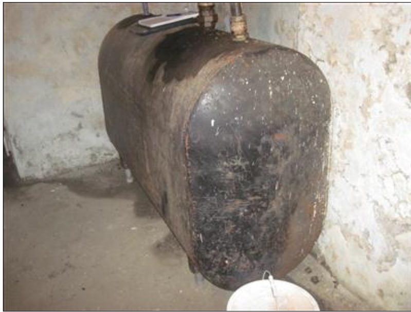
G. Picture 3 second tank in basement
