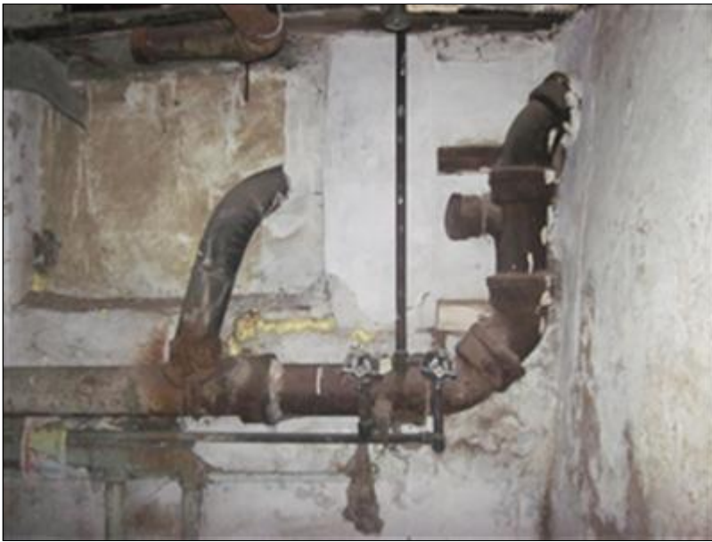
B. Picture 3 leaking / corroded drains
