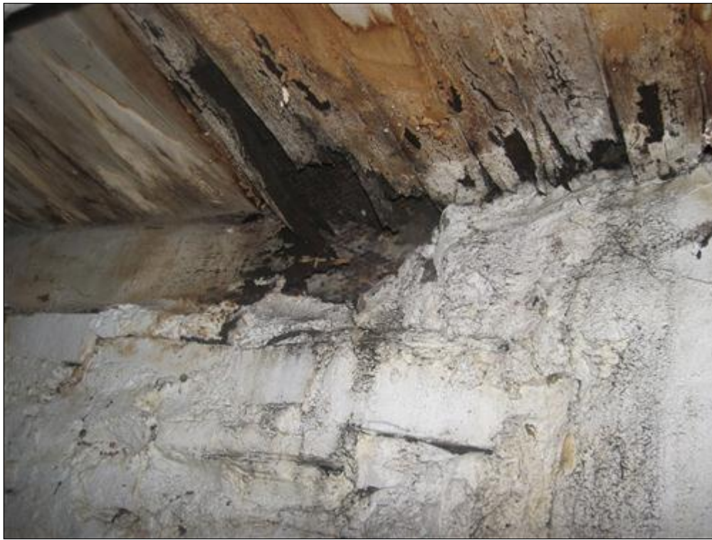
B. Picture 3 rot/termite damage
