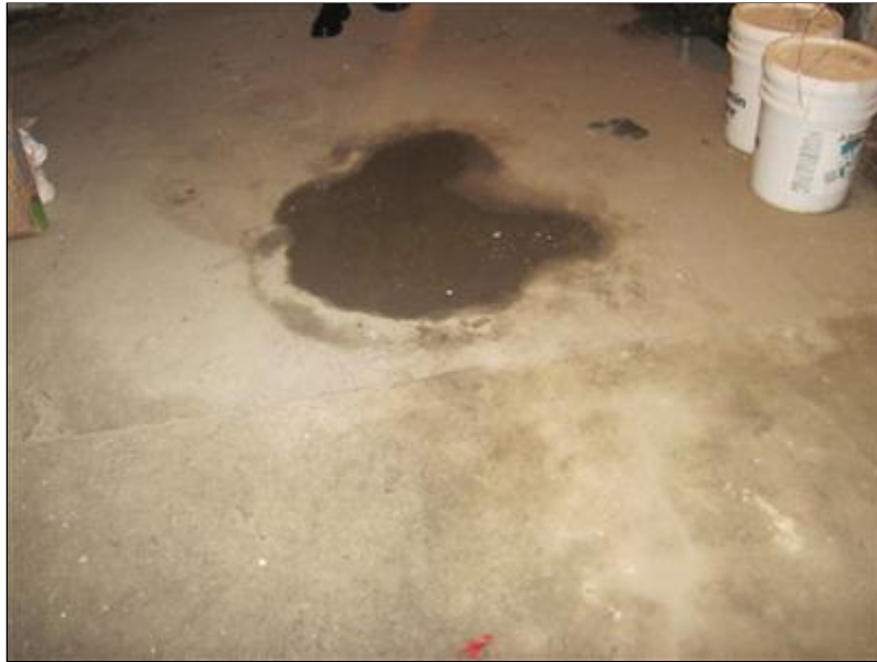
A. Picture 1 wet basement / water entry
