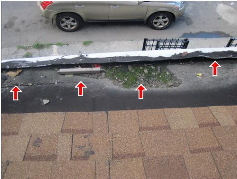
D. Picture 1 open joints/deteriorated roof
