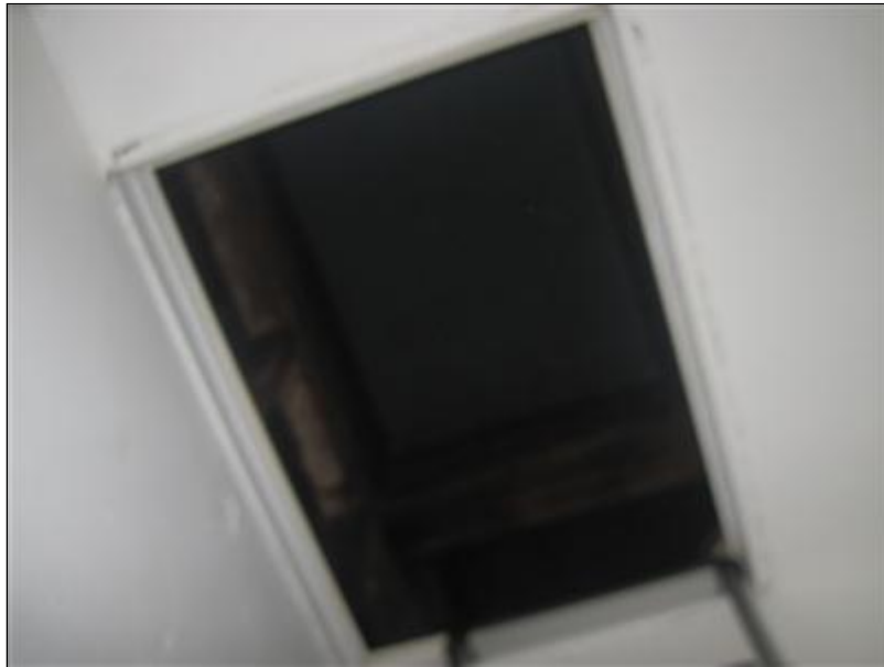
E. Picture 2 sealed roof opening
