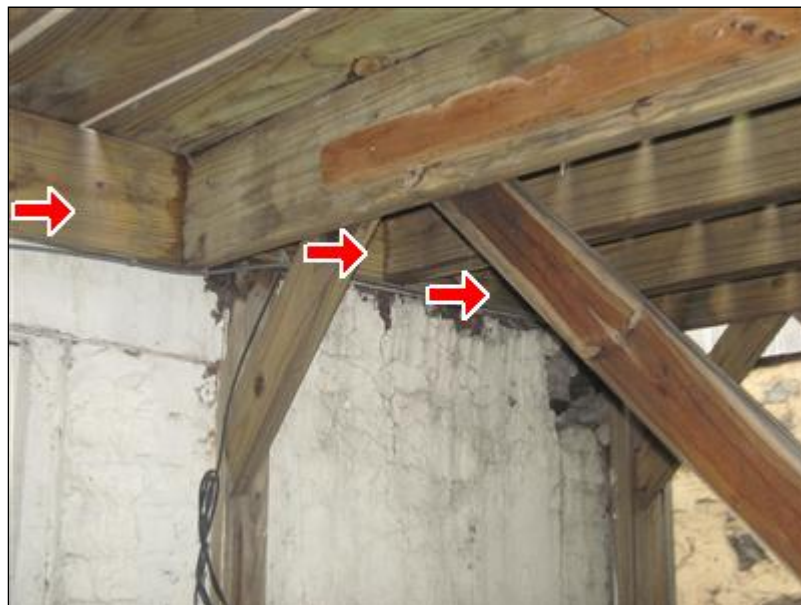
K. Picture 4 missing anchor bolts
