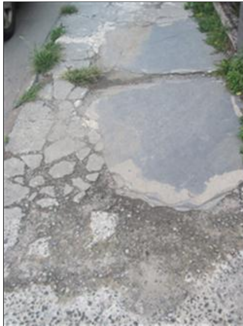
C. Picture 3 cracked / deteriorated sidewalks
