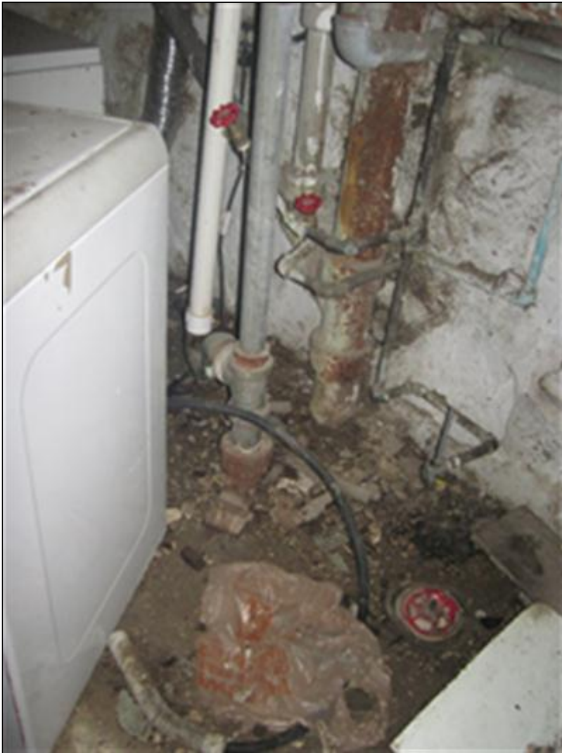
B. Picture 4 leaking corroded drains
