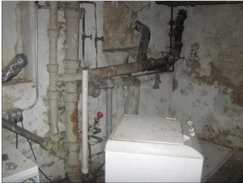
B. Picture 1 corroded / leaking drains
