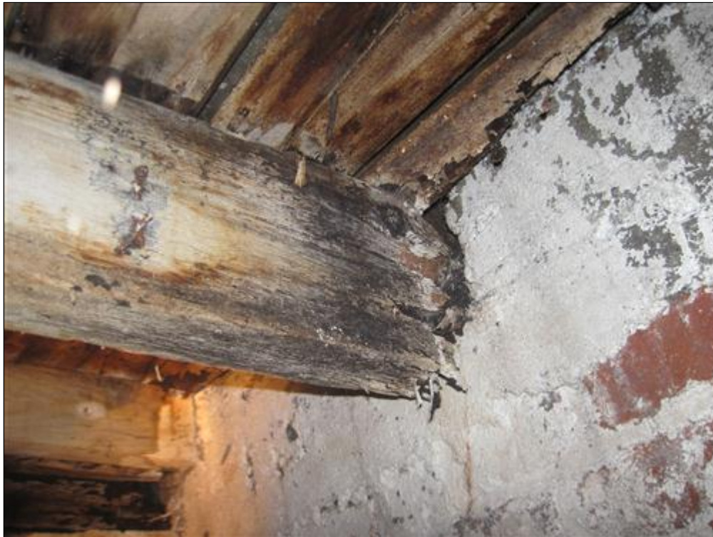
K. Picture 2 collapsing support joist
