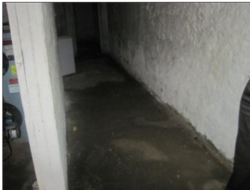
A. Picture 4 wet basement
