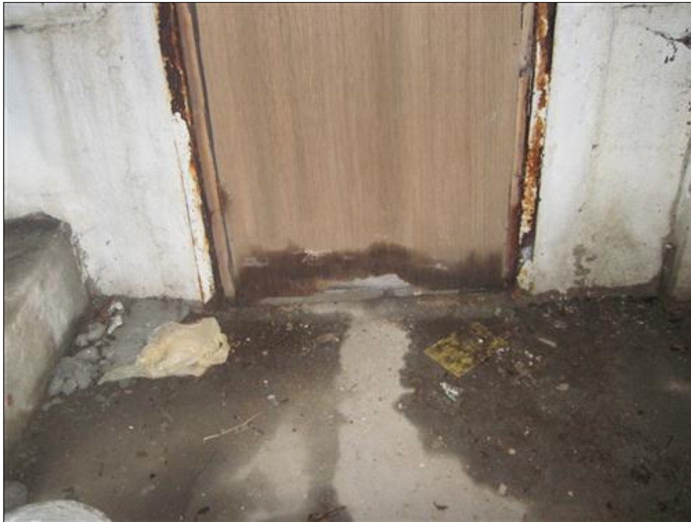
A. Picture 2 water entry in basement
