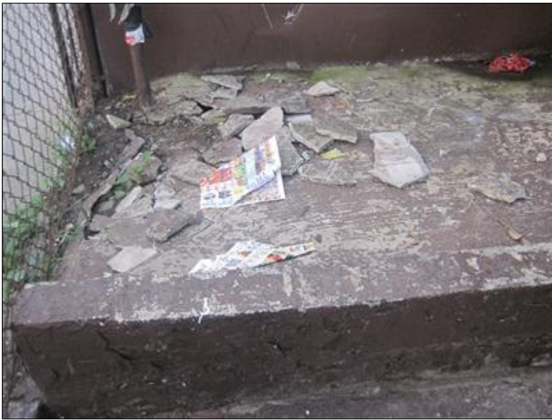
C. Picture 5 broken concrete / buried tank
