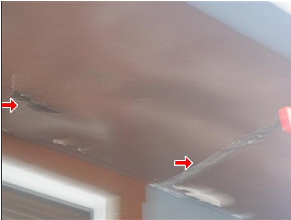
K. Picture 3 leak / damage
