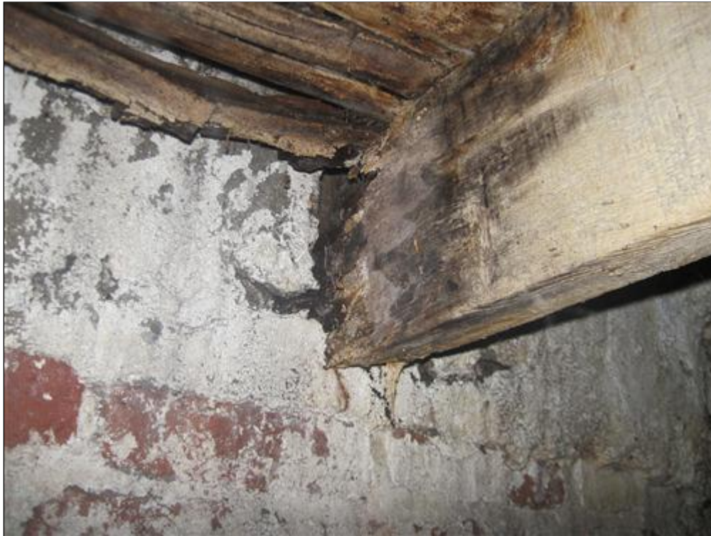
K. Picture 1 collapsing support joist
