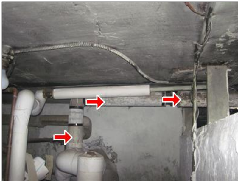
G. Picture 4 Asbestos insulation
