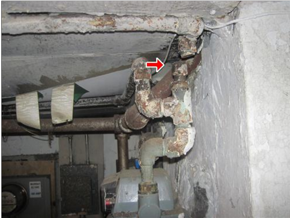
G. Picture 1 disconnected gas line/meter
