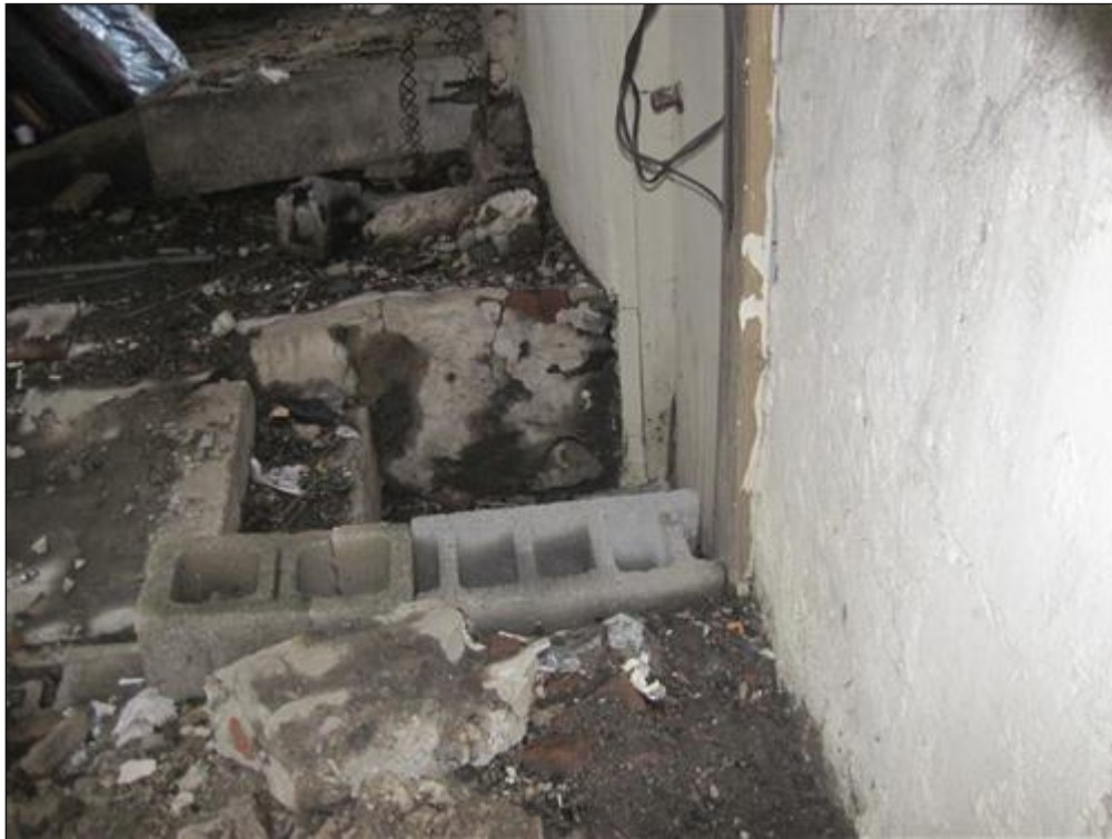
C. Picture 2 water entry / damage
