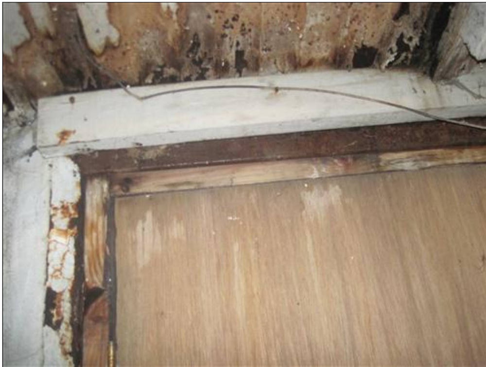
B. Picture 5 extensive damage
