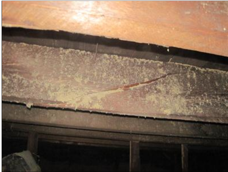
E. Picture 1 cracked rafter
