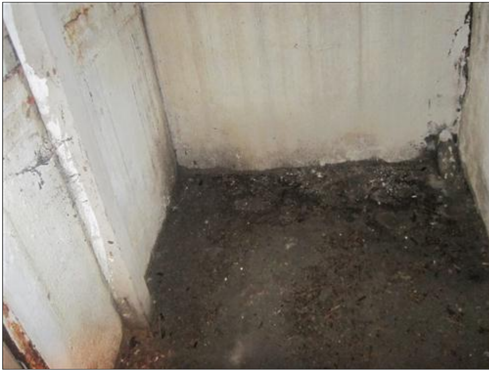
A. Picture 3 wet basement
