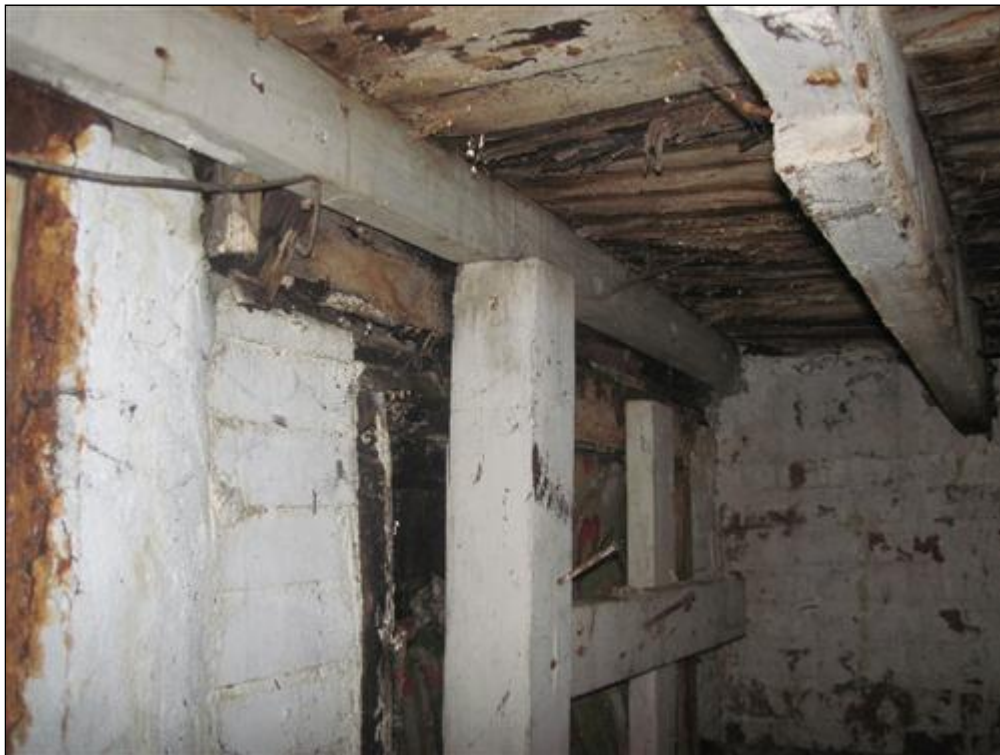
B. Picture 4 collapsing front entire area
