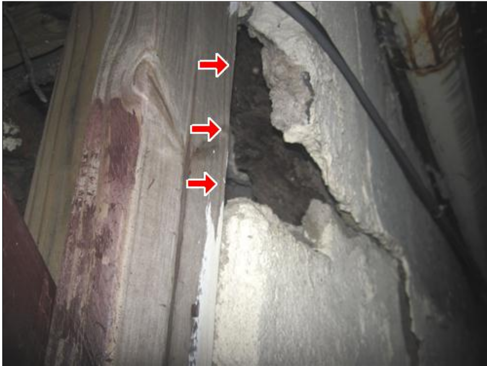
B. Picture 1 rot / termite damaged structural framing
