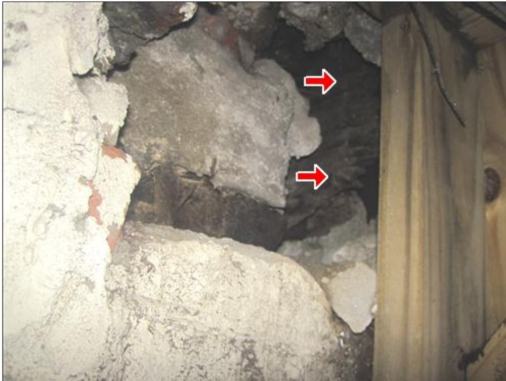
B. Picture 2 rot/termite damaged framing
