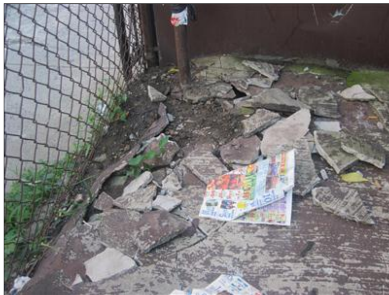
C. Picture 4 broken concrete
