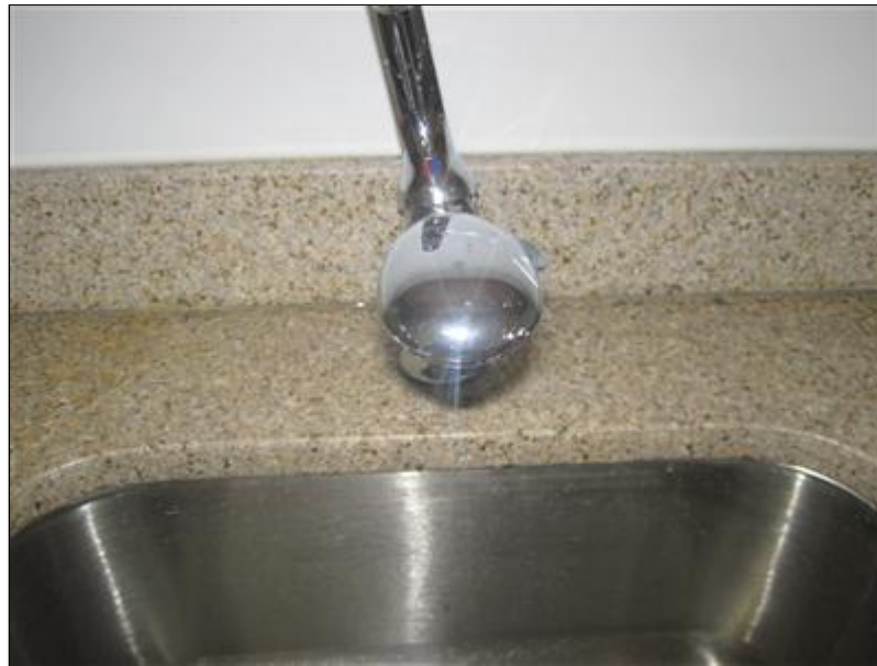
A. Picture 1 loose fixture
