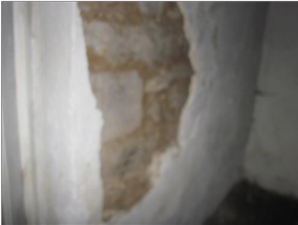
A. Picture 5 moisture damage
