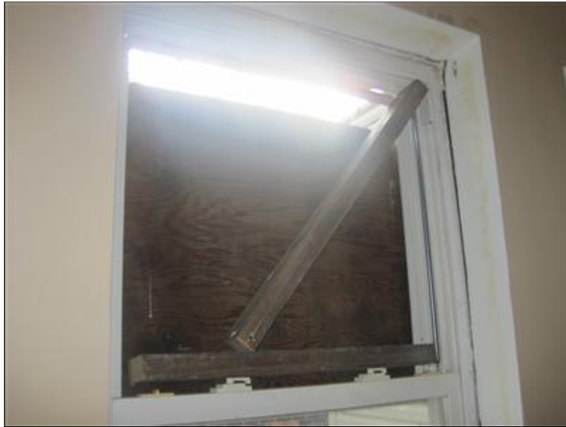
I. Picture 1 broken / missing window
