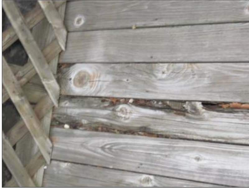
K. Picture 3 rot damage
