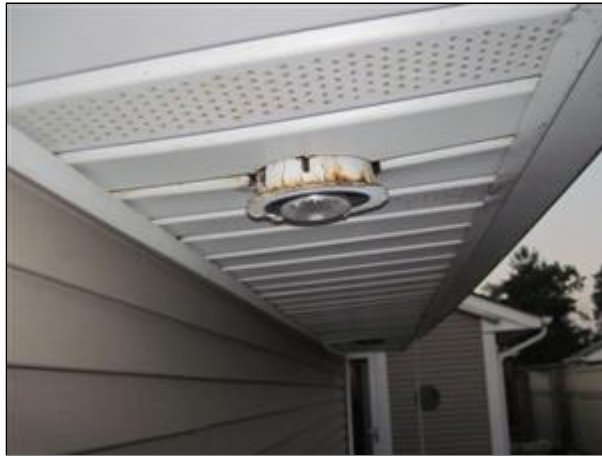
D. Picture 8 leak from roof
