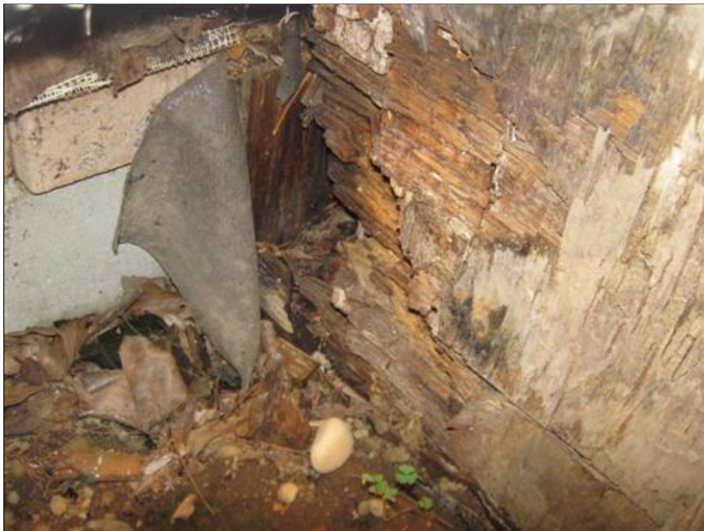
F. Picture 2 rot damage wood framing
