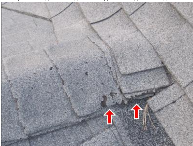
D. Picture 1 crumbling shingles
