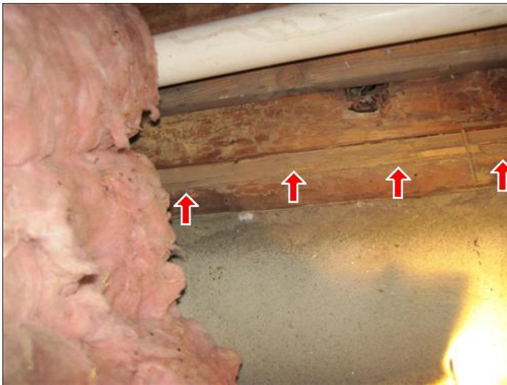
F. Picture 7 termite damage
