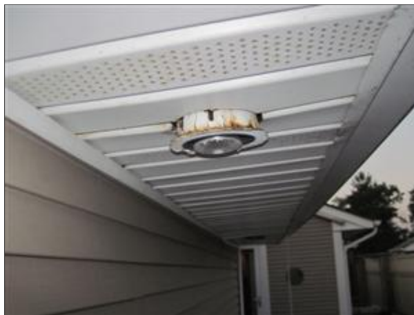
D. Picture 8 leak from roof
