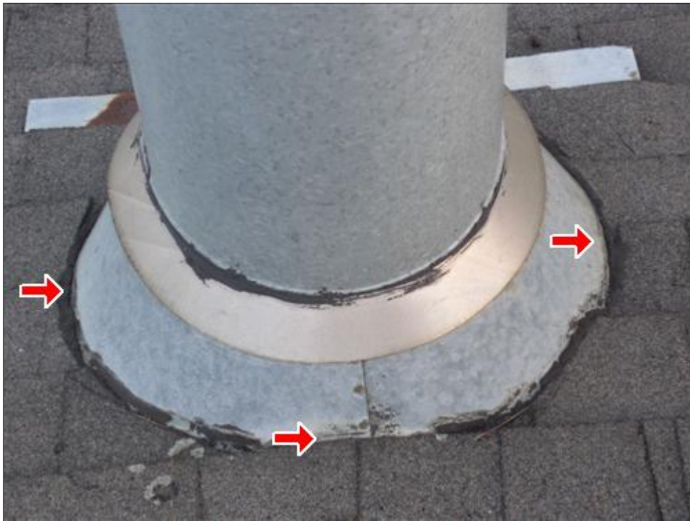
D. Picture 5 open joint / missing sealer
