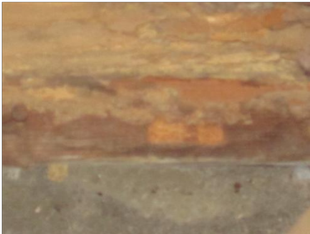
F. Picture 8 termite damage
