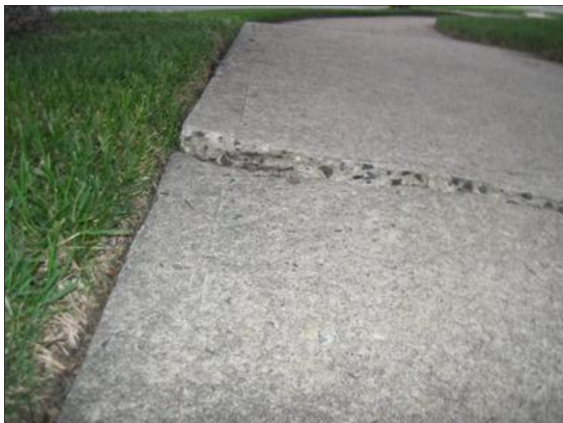
C. Picture 3 broken / cracked concrete sidewalk
