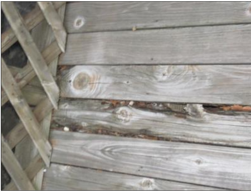
K. Picture 3 rot damage
