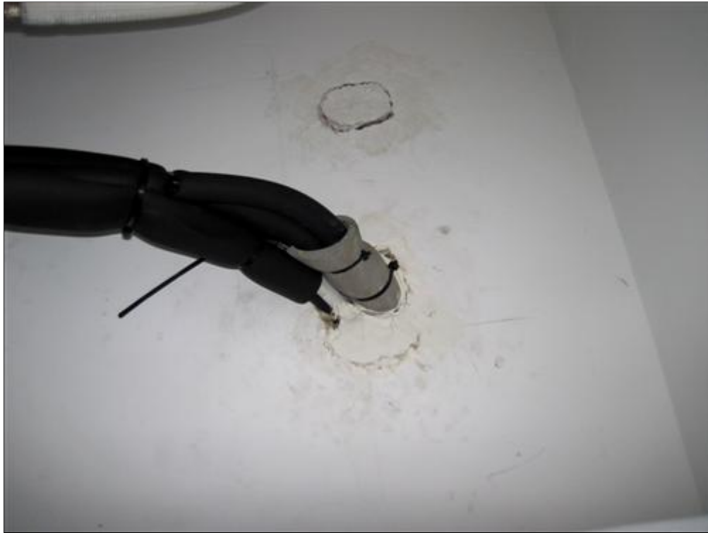
G. Picture 1 moisture leak
