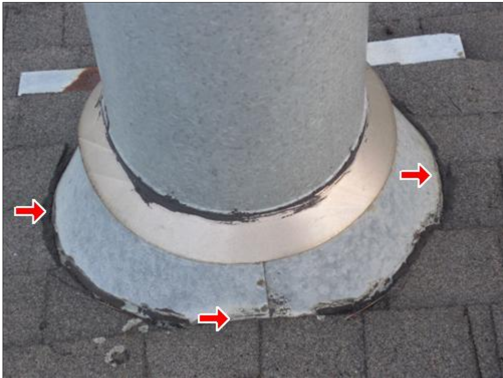
D. Picture 5 open joint / missing sealer
