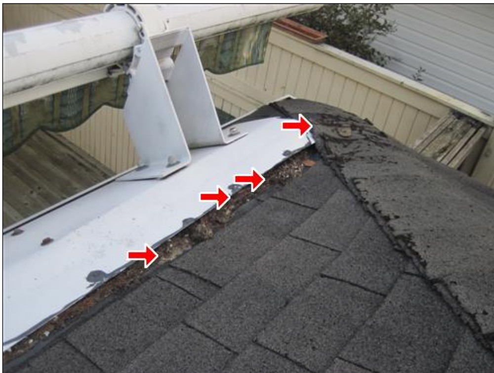
D. Picture 6 debris filled area / poor flashing
