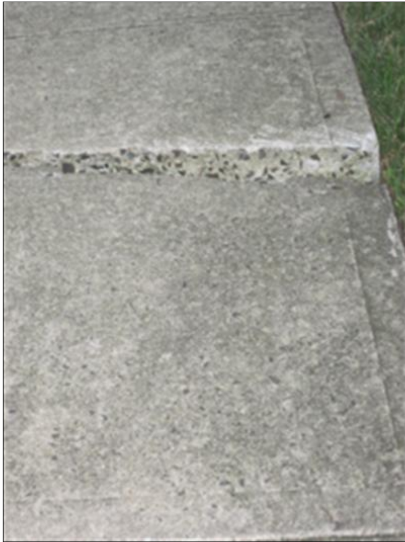
C. Picture 2 cracked sidewalk
