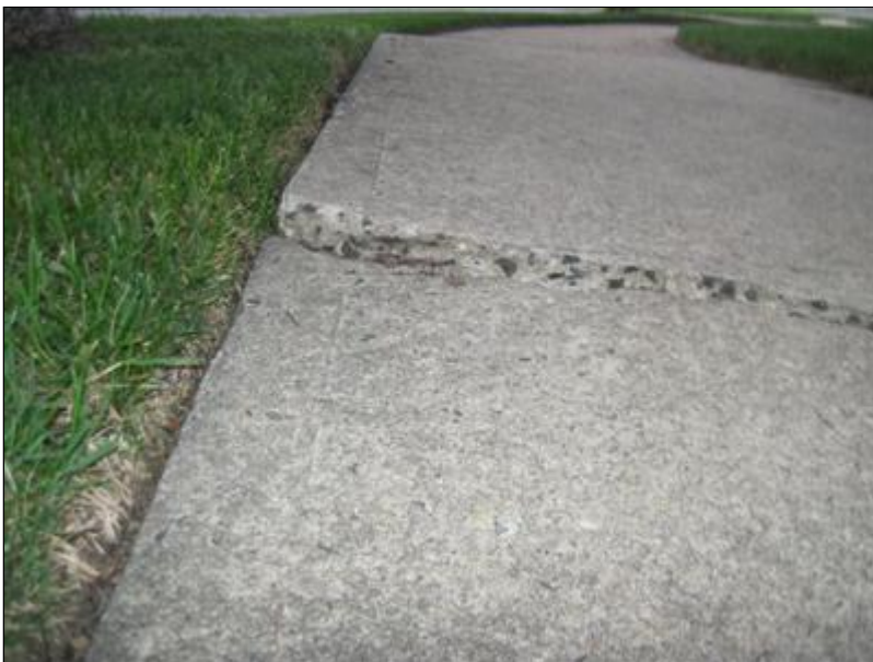
C. Picture 3 broken / cracked concrete sidewalk
