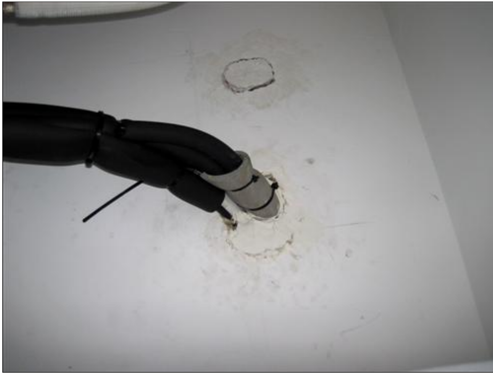
G. Picture 1 moisture leak
