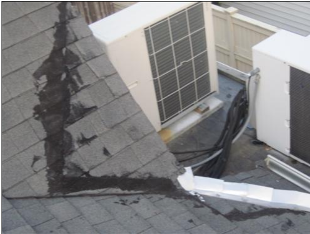
D. Picture 3 poor repair / workmanship
