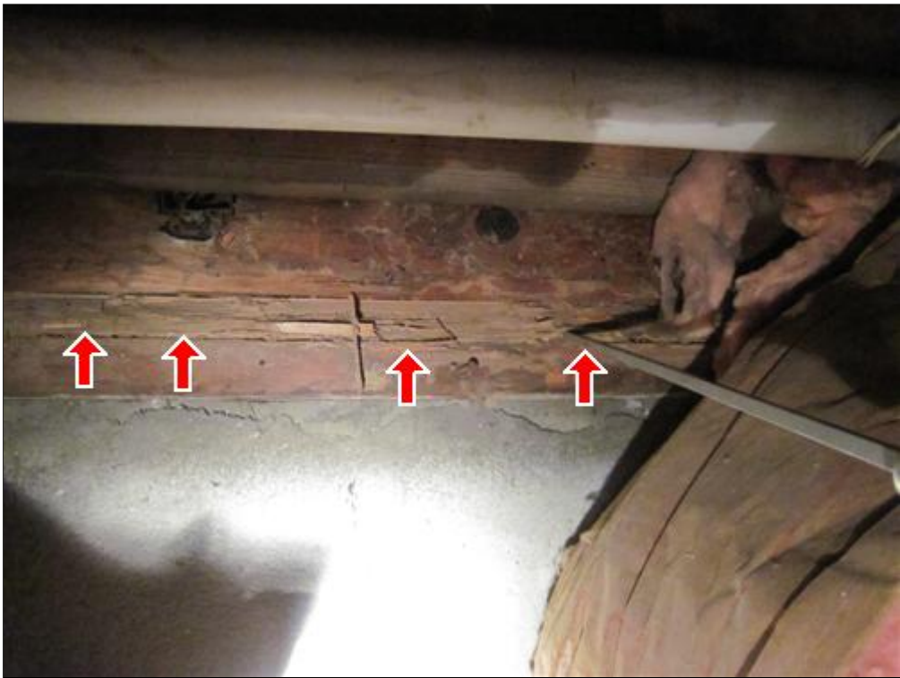
F. Picture 6 termite infestation / damage
