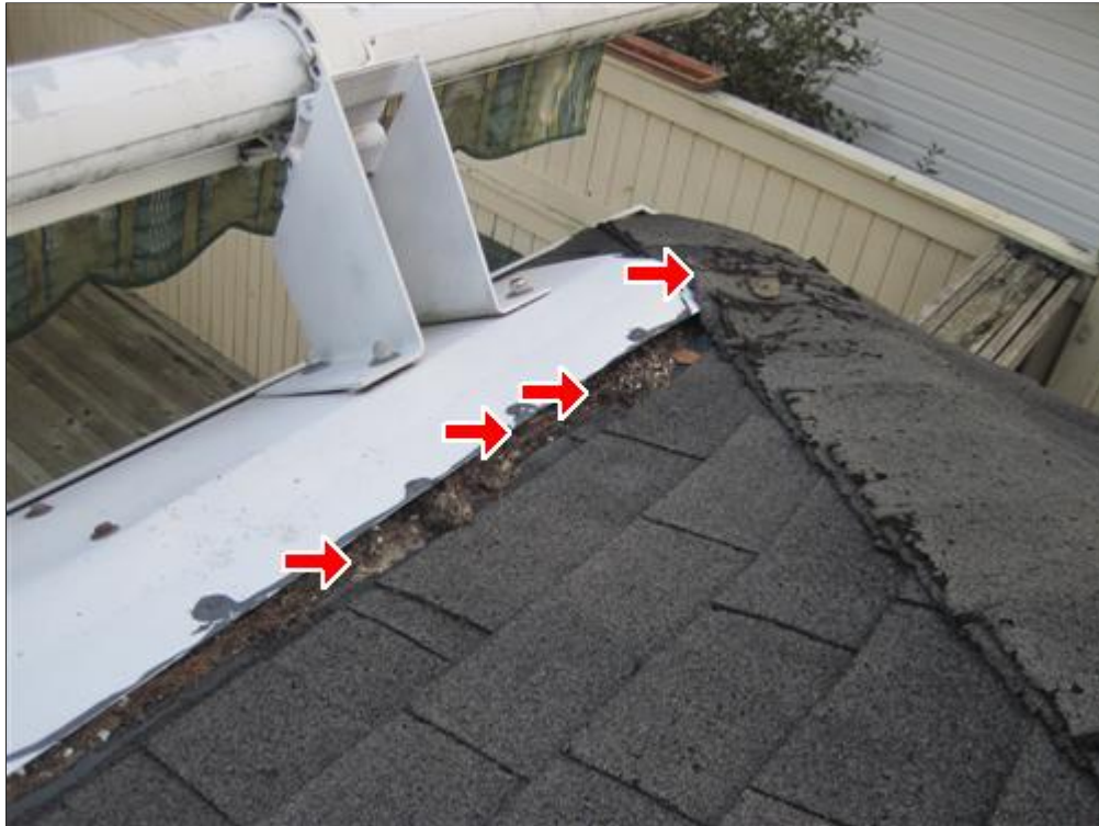
D. Picture 6 debris filled area / poor flashing
