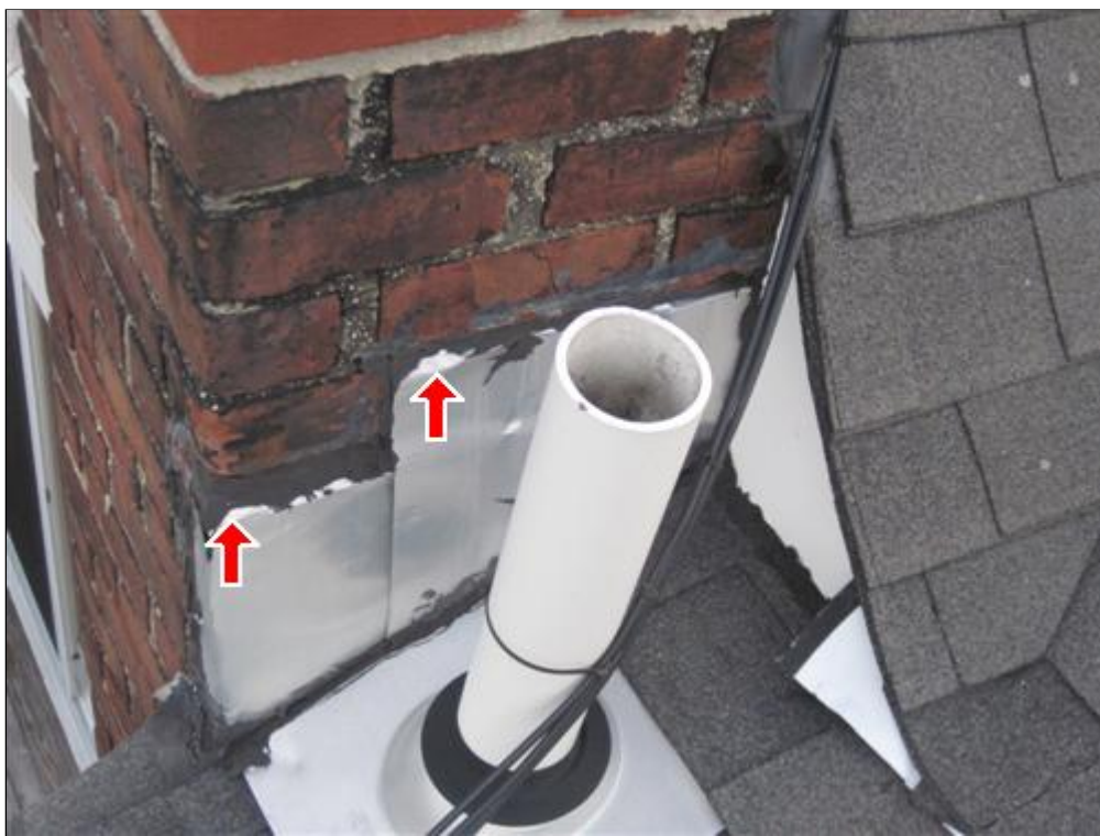
J. Picture 2 poor sealing / workmanship
