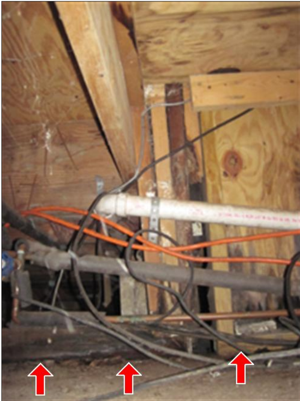
K. Picture 5 water entry / damage
