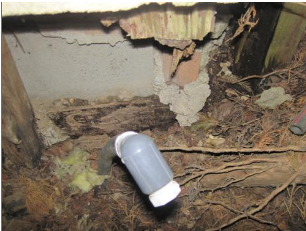
F. Picture 3 rot damage
