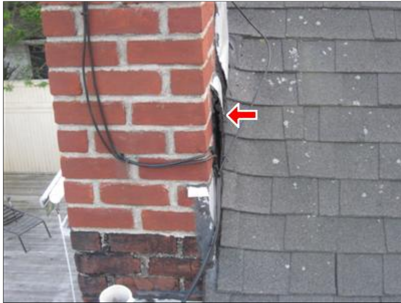
J. Picture 1 open joints
