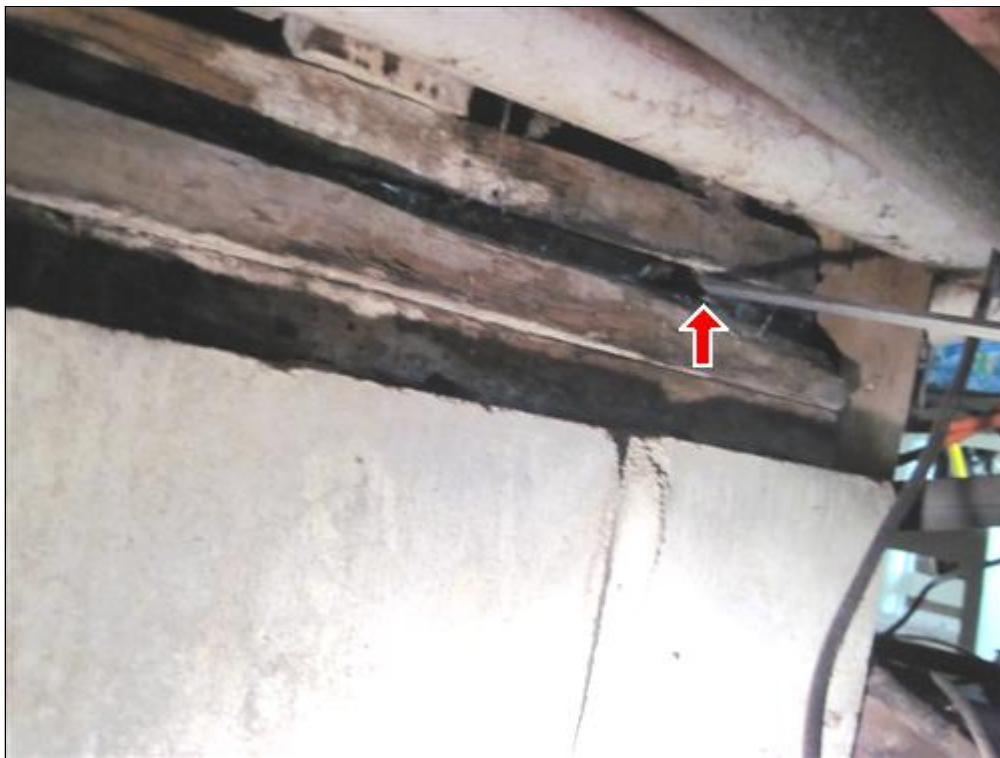
F. Picture 5 damaged sill
