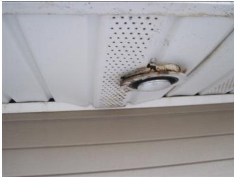
D. Picture 7 corroded light fixture from leak
