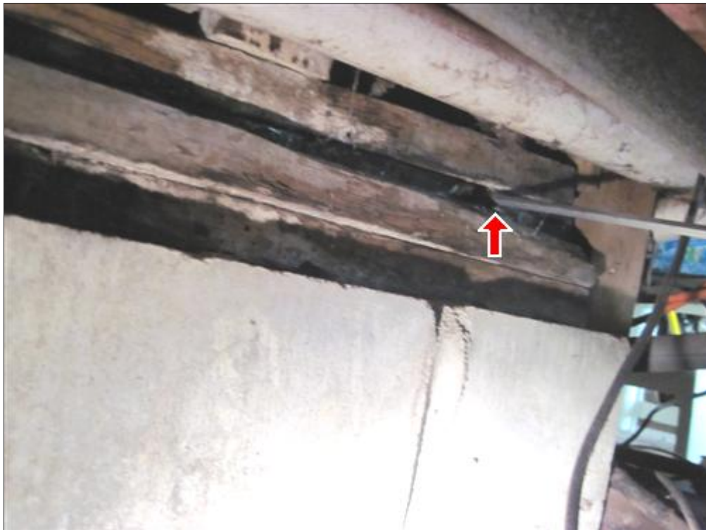
F. Picture 5 damaged sill
