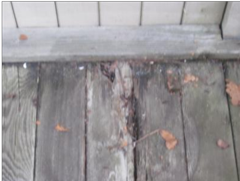
K. Picture 2 rot damage
