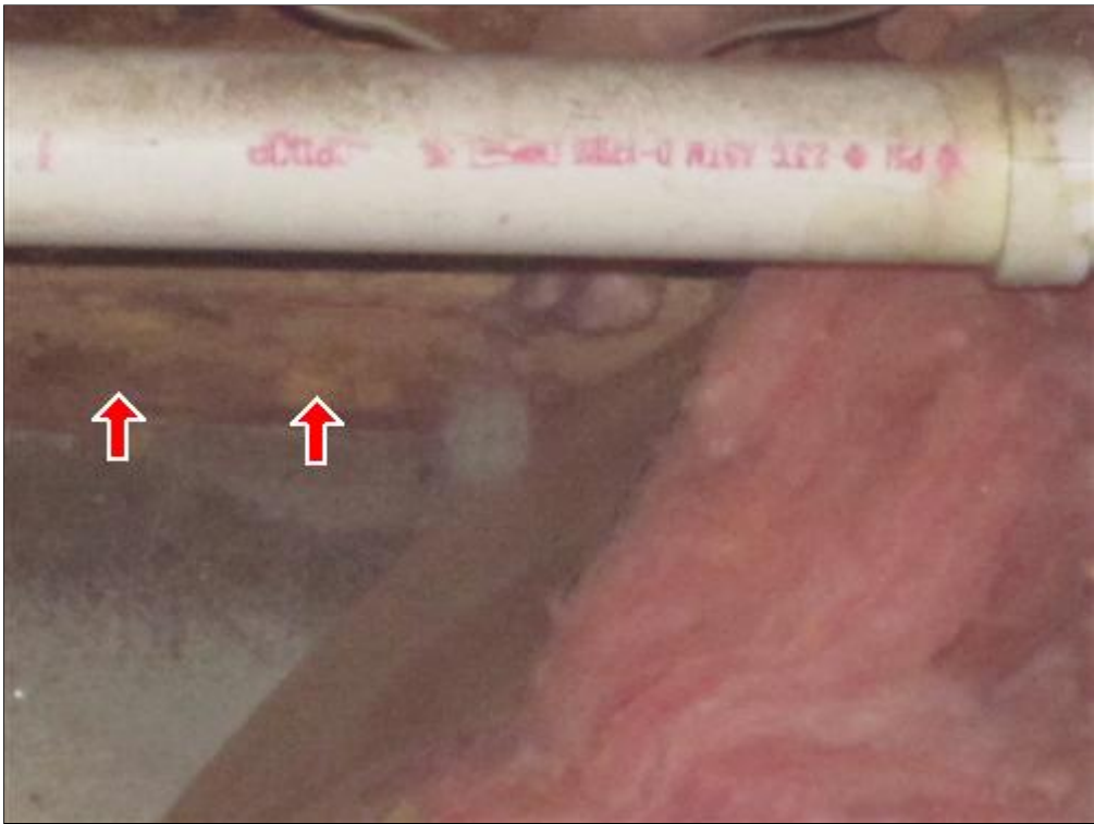
K. Picture 6 possible water damage at end of crawl space
