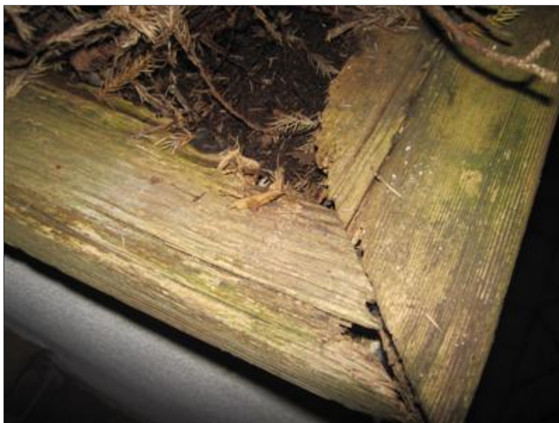
C. Picture 4 rot damaged wood
