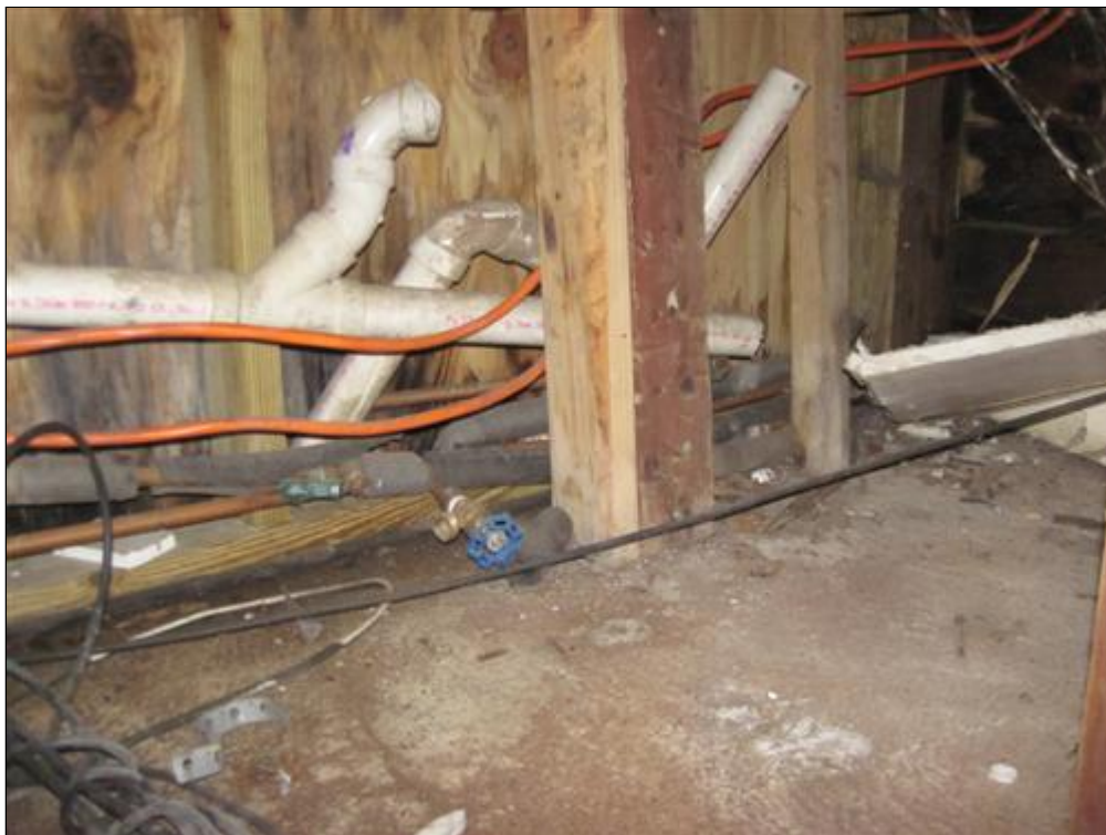
K. Picture 8 moisture entry, abandoned drains, rot
