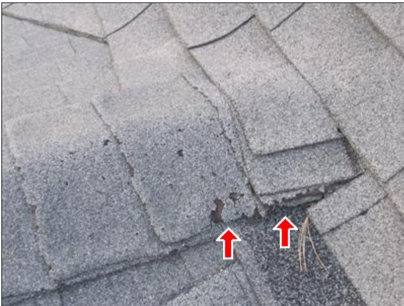
D. Picture 1 crumbling shingles
