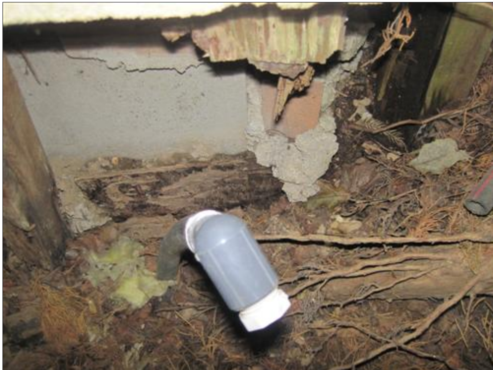
F. Picture 3 rot damage
