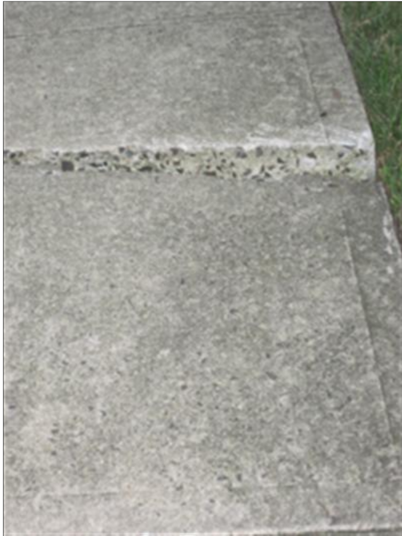
C. Picture 2 cracked sidewalk
