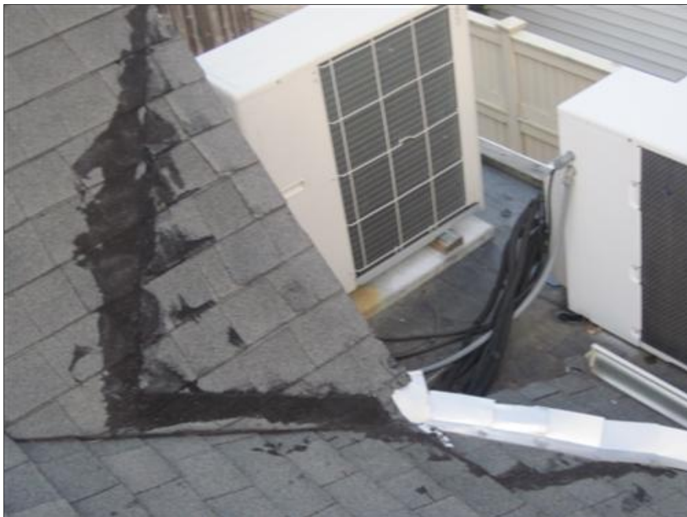
D. Picture 3 poor repair / workmanship
