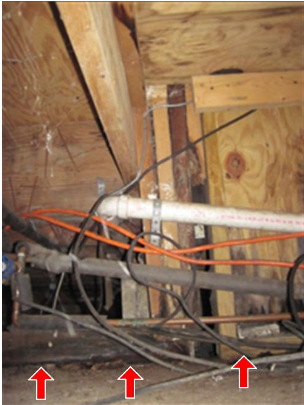
K. Picture 5 water entry / damage
