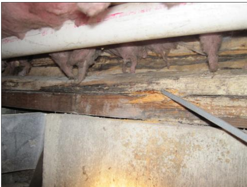
F. Picture 4 damaged sill
