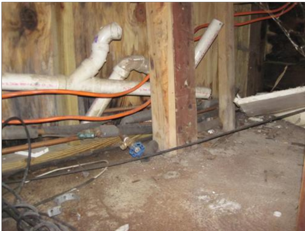
K. Picture 8 moisture entry, abandoned drains, rot
