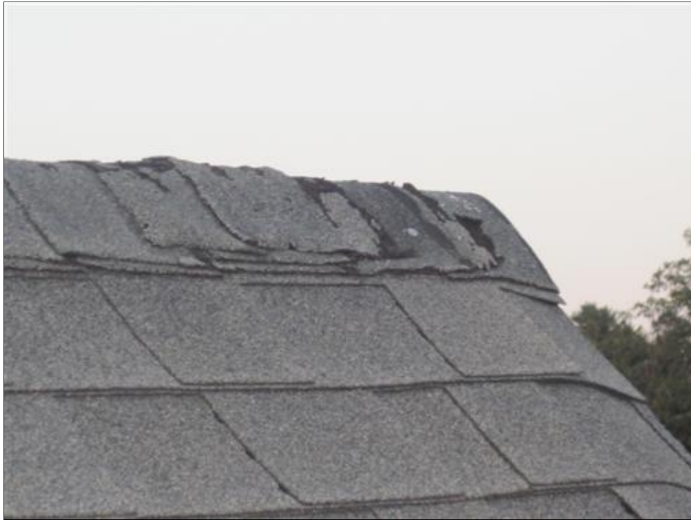
D. Picture 4 deteriorated ridge shingles
