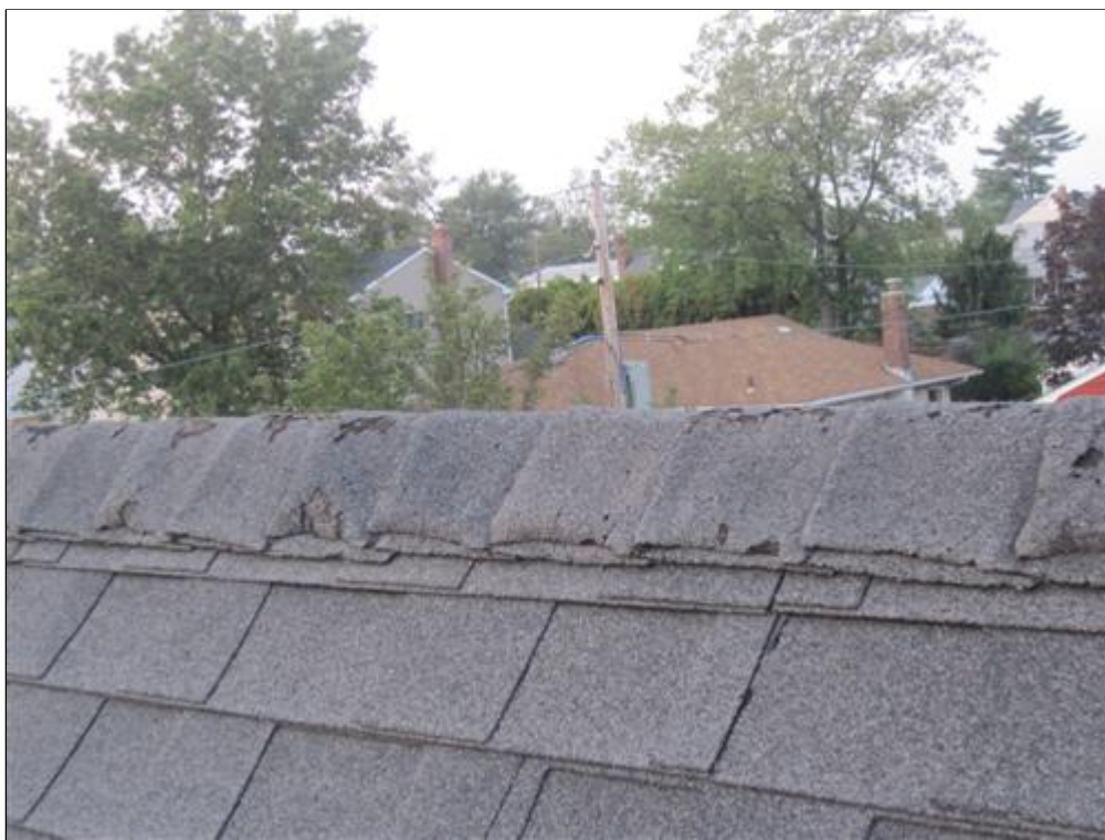
D. Picture 2 warped / crumbling shingles
