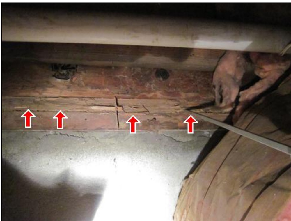
F. Picture 6 termite infestation / damage
