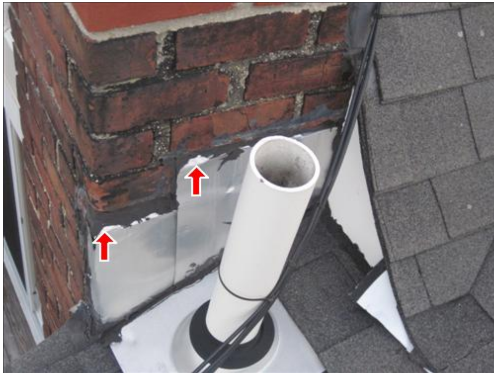
J. Picture 2 poor sealing / workmanship
