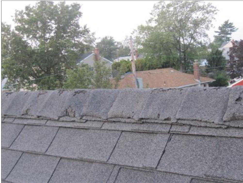
D. Picture 2 warped / crumbling shingles
