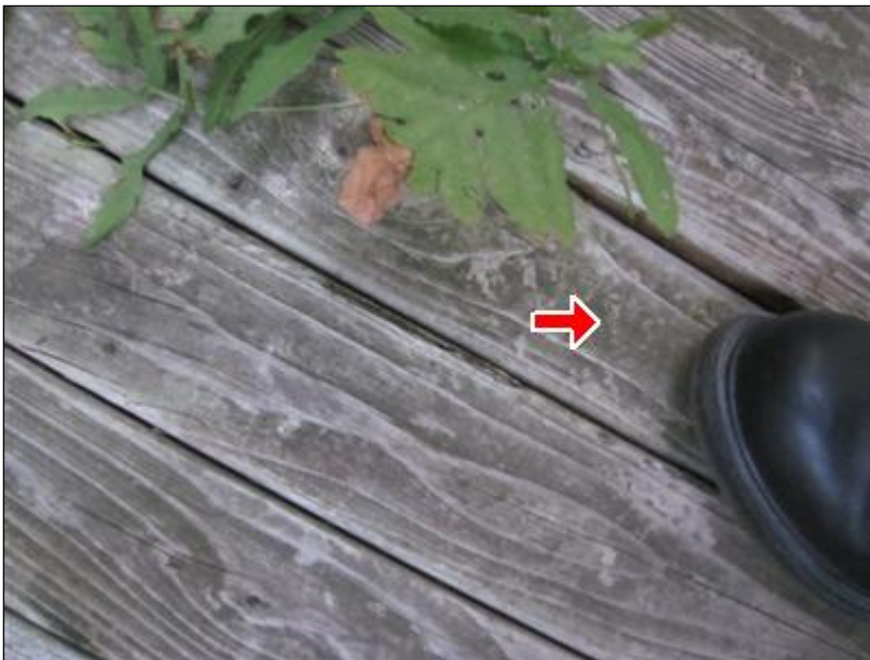
K. Picture 1 collapsing board
