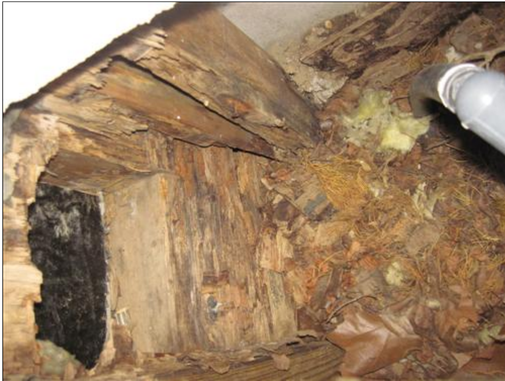
F. Picture 1 rot damage
