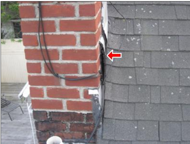
J. Picture 1 open joints
