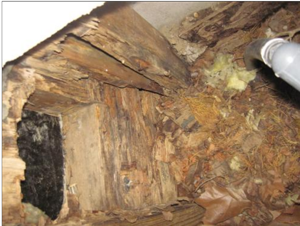
F. Picture 1 rot damage
