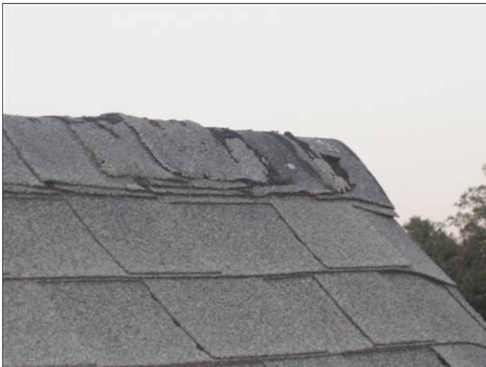
D. Picture 4 deteriorated ridge shingles
