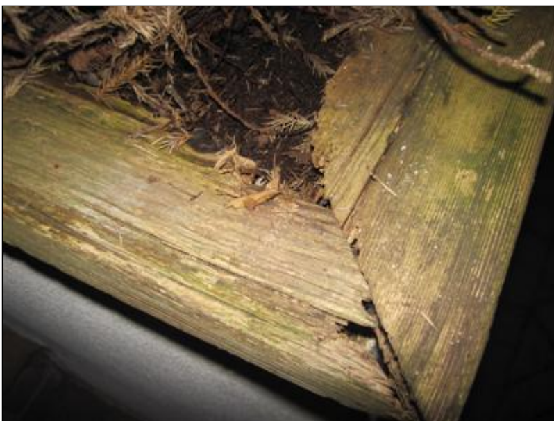
C. Picture 4 rot damaged wood
