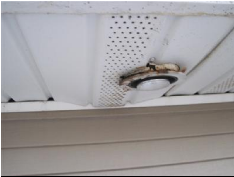
D. Picture 7 corroded light fixture from leak
