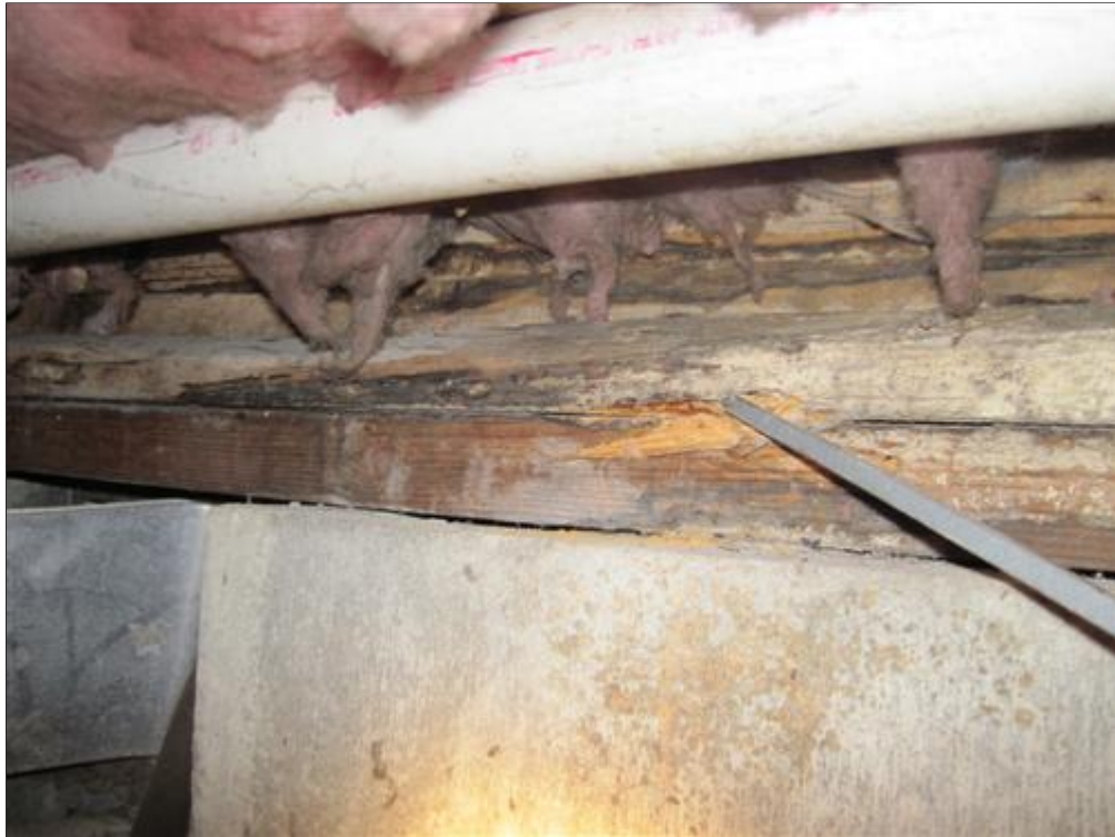
F. Picture 4 damaged sill
