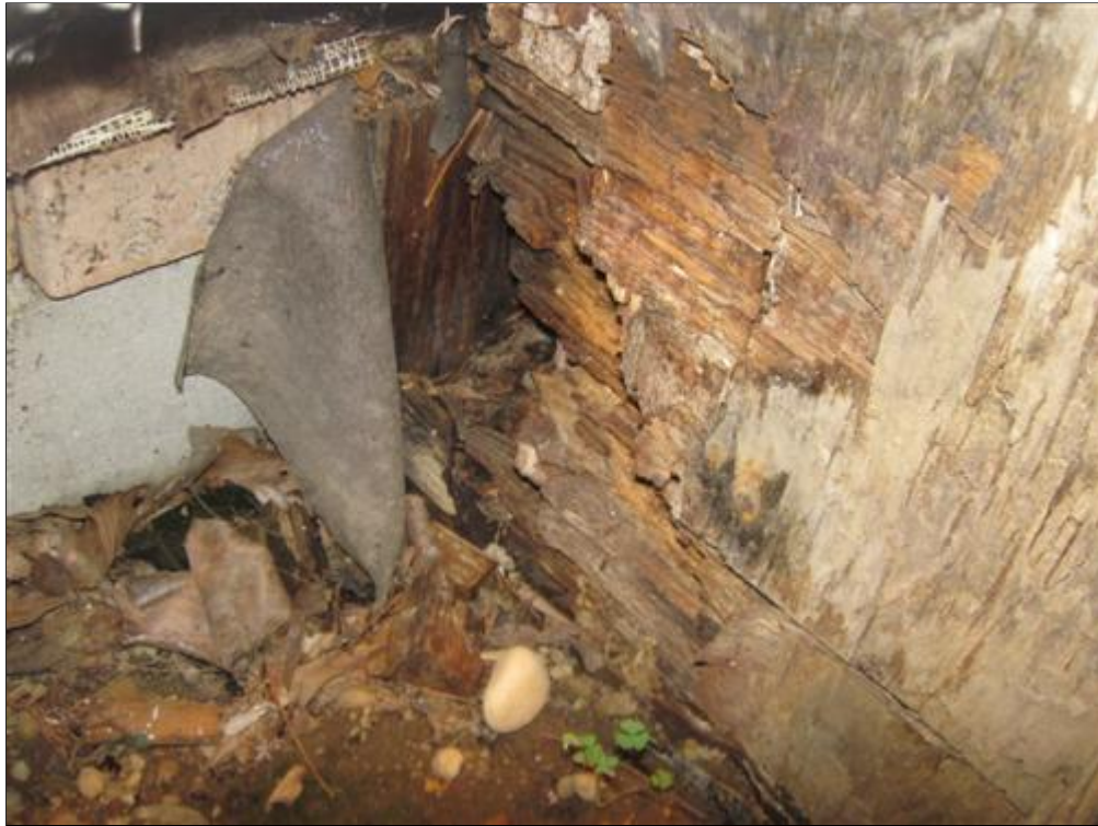
F. Picture 2 rot damage wood framing
