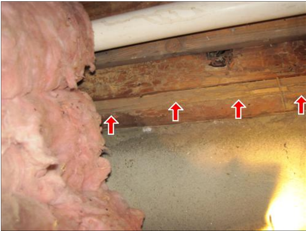
F. Picture 7 termite damage
